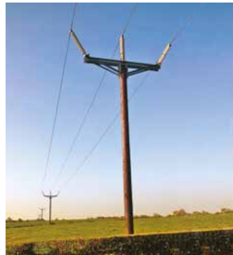
Single wood pole Trident – approx. 12m
